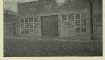
GARAGE OF J. W. CHENOWORTH, ALBANY, MO.
