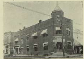
BANK OF ALBANY, ALBANY, MO.
